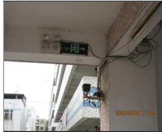
Photo of the dormitories (if applicable) Fire exit sign and emergency lights at dormitory building.JPG
