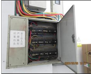
Photo of non-conformity The inner protective board of two sampled electronic boxes were missed 1.JPG
