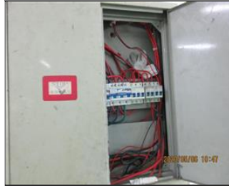
Photo of non-conformity The inner protective board of two sampled electronic boxes were missed 2.JPG
