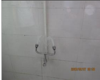
Photo first aid facilities Eye washing facility.JPG
