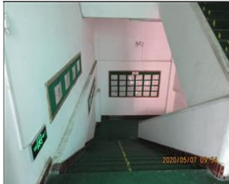
Photo of fire safety equipment Emergency lights and evacuation indication sign in fire stair.JPG
