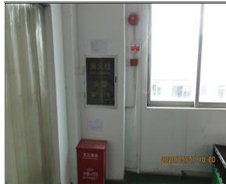
Photo of fire safety equipment Fire extinguishers and fire hydrant and fire alarm button.JPG
