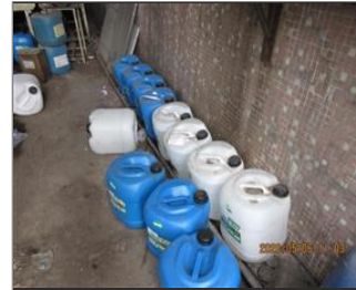
Photo of non-conformity No suitable prevent leakage secondary containment was installed for the chemical in chemical stored.JPG
